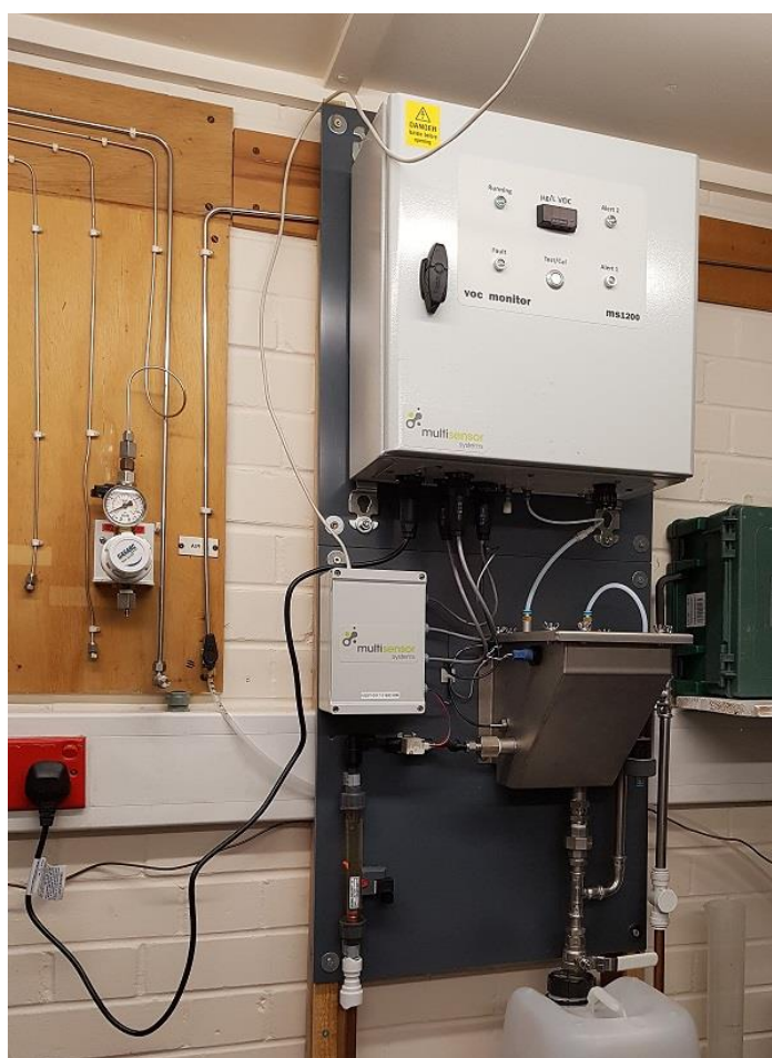
Figure 15 - A picture of the unit installed in the outbuilding. The unit is connected to a PLC that records the data and, in case of an accident, triggers an alarm that switches off the intake pumps.
