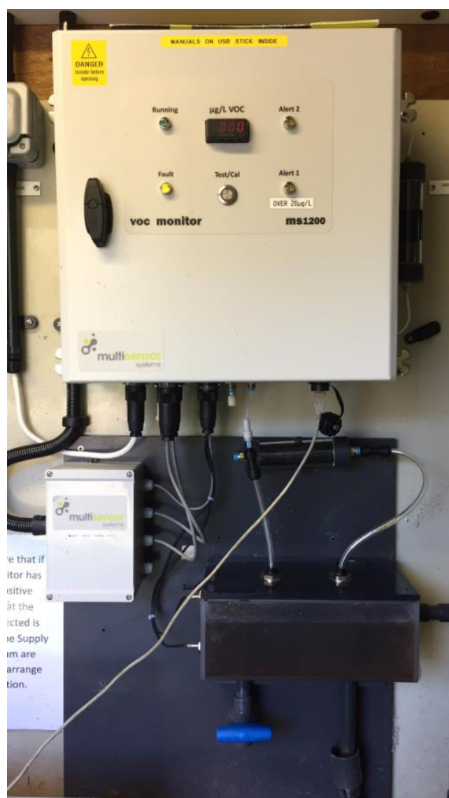
Figure 16 - A picture of the unit installed in the outbuilding. The unit controls a sluice gate which diverts flow away from the reservoir in the event of contamination
